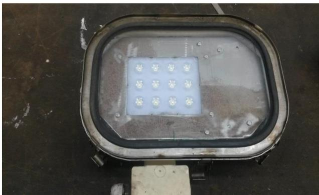
Replace the glass and lock it with the clamps. Screw the connection box together.
