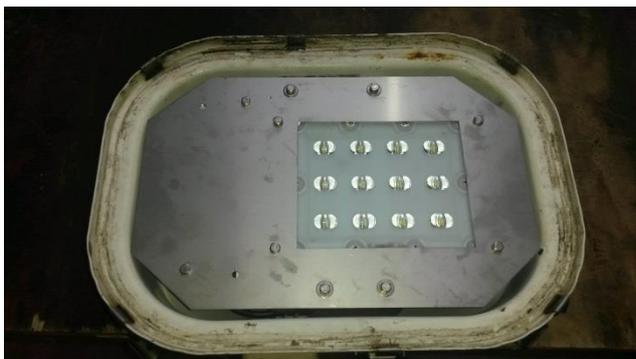
Place the module plate in the fixture and screw it tight with the included M4x10 + lock washer and fender washer.
