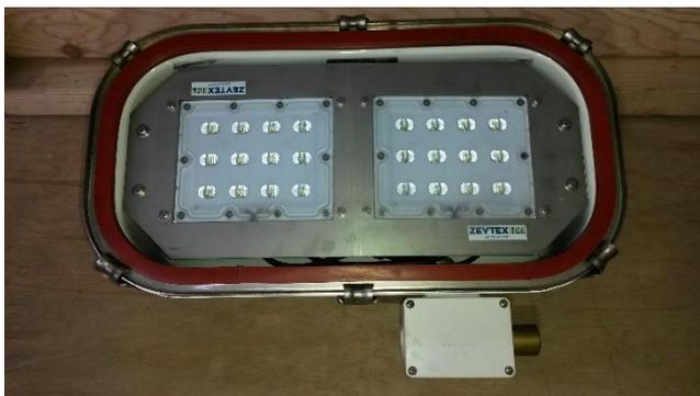
Replace the glass and lock it with the clamps. Screw the connection box together.
