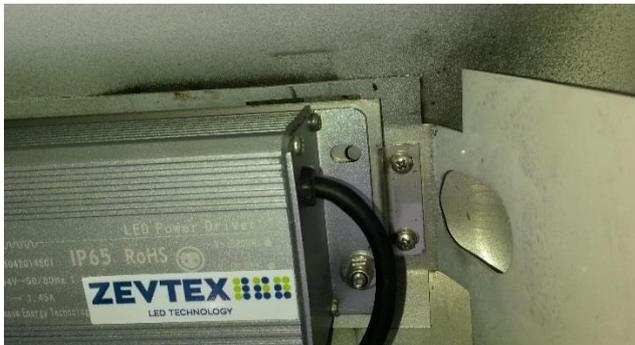
Attach the driver plate on the bottom of the fixture in the existing screw holes with the supplied M3x8 + lock washer.
