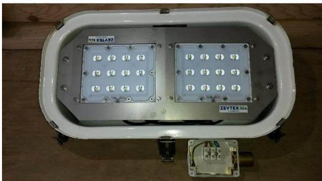
Place the module plate in the fixture and screw it tight in the existing screw holes with the supplied M4x10 + lock washer and fender washer.
