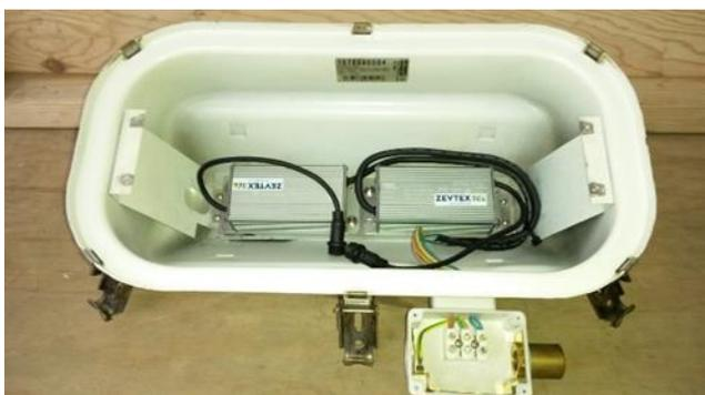
Attach the wiring in the connection box (if you wish, you can use the supplied terminal block). Fix the wiring with the tie-wrap.
